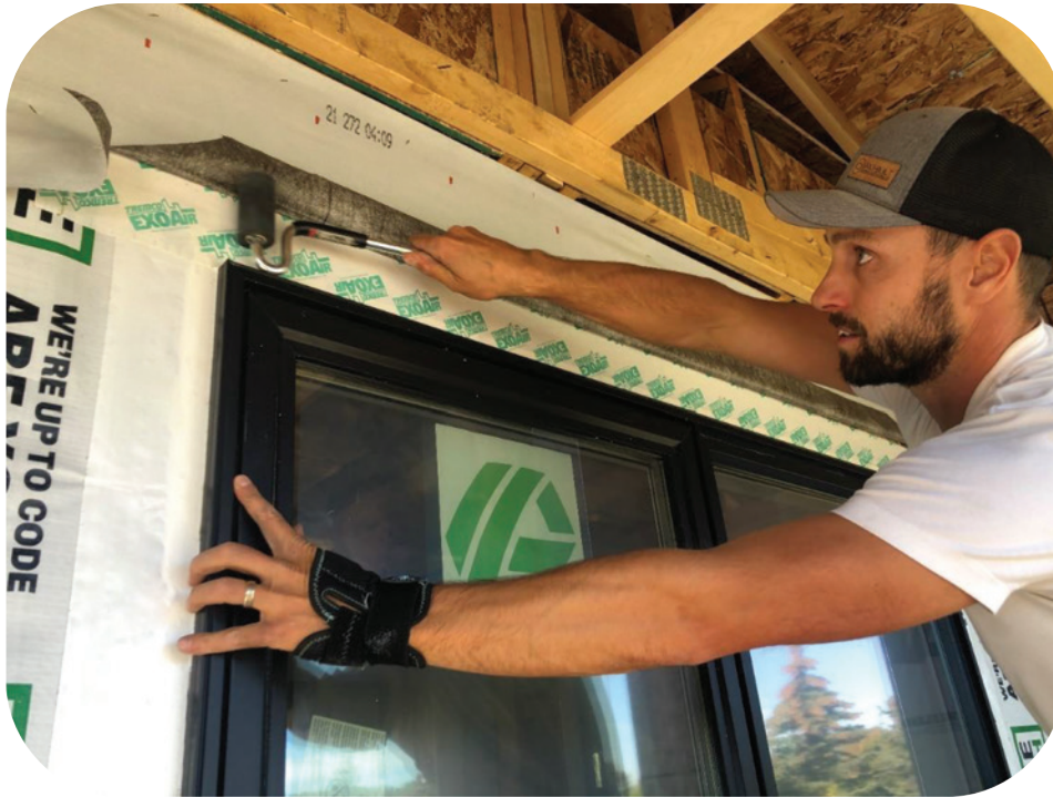
Apply flash tape above the window and onto the substrate above ensuring tape over vertical flashings using a J Roller.
