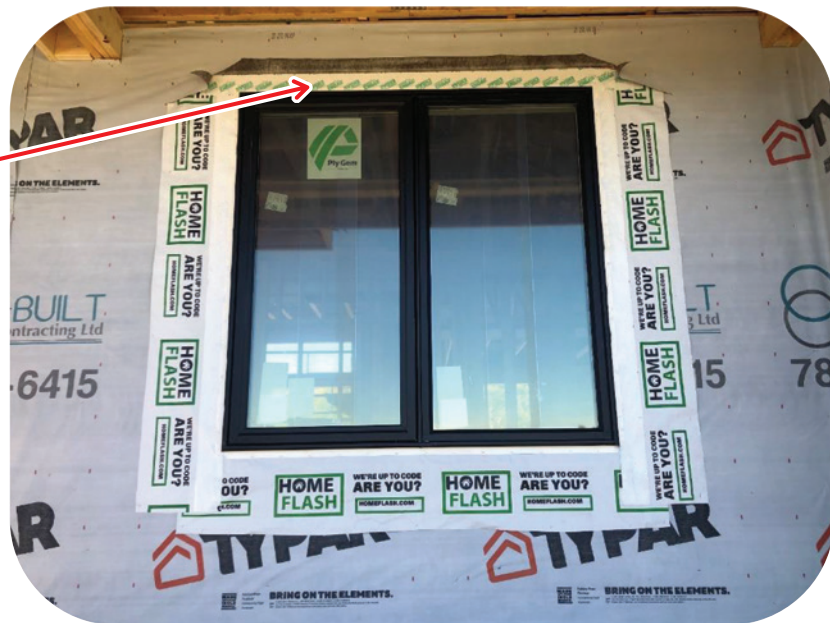
Apply flash tape above the window and onto the substrate above ensuring tape over vertical flashings using a J Roller.
