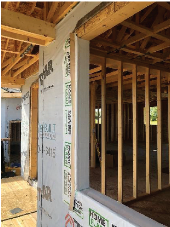
Fasten the jamb flash over the WRB with tacker stapler.
